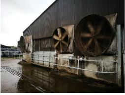
The main livestock housing sheds houses 250 number of cattle and is specialist designed with polycarbonate sheeting surrounding reducing the UV penetration that would otherwise (with conventional clear plastic cladding) causing a greenhouse effect in the building. The building and is designed to provide 16 hours of light which,
